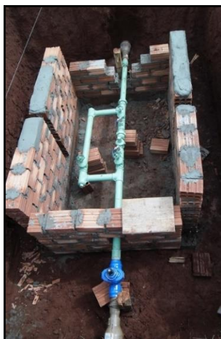
Figure 5 – Shelter for the installation of a direct acting PRV
