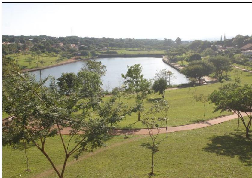
Figure 2 – Detention basin located in the park Alfredo Werner Nyffeler, in Maringá - PR
