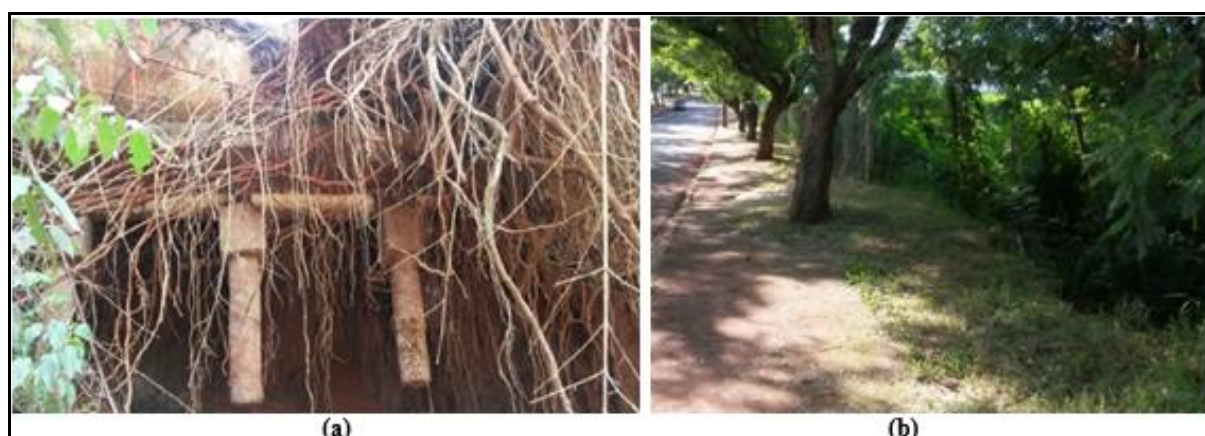
Figure 4 – Erosive process downstream the park Alfredo Werner Nyffler
