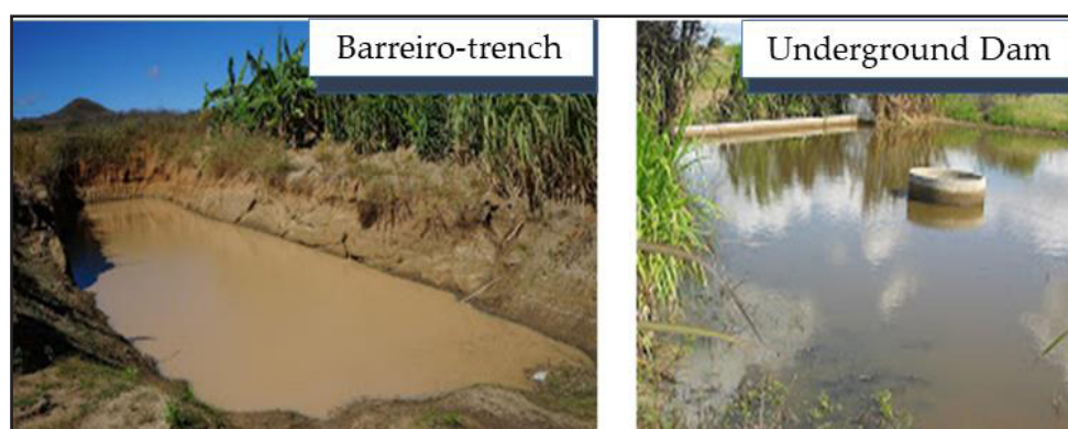
Figure 8 – Barreiro trench 5 and underground dam 6
