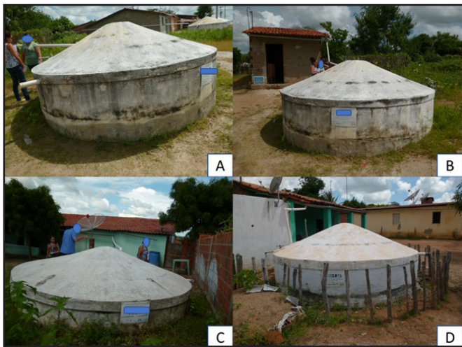
Figure 10 – Plate cisterns (A, B, C and D) in the municipality of Ibaretamas, Sertão Central, Ceará.
