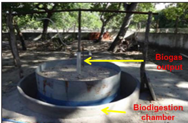
Figure 2 – Indian biodigester, community of Uruá, municipality of Barreira, Baturité Massif, Ceará
