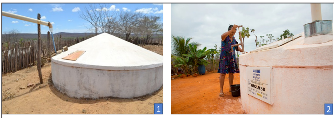
Figure 6 – Cisterns for human consumption of 16 thousand liters 1,2 .
