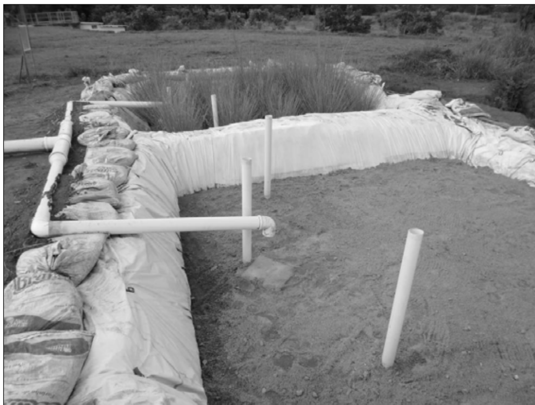
Figure 1 - General view of the experimental septic waste treatment plant built
